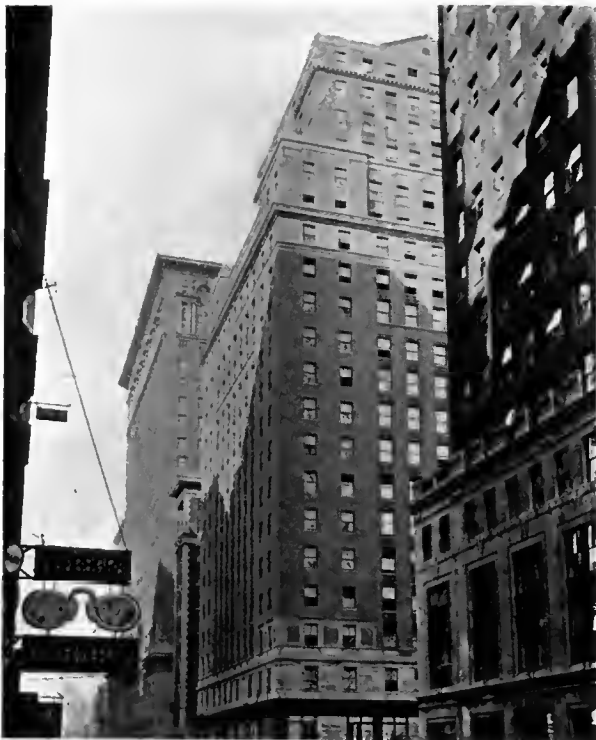
FIG. 3. LIGGETT BUILDING, FORTY-SECOND STREET, NEW YORK
